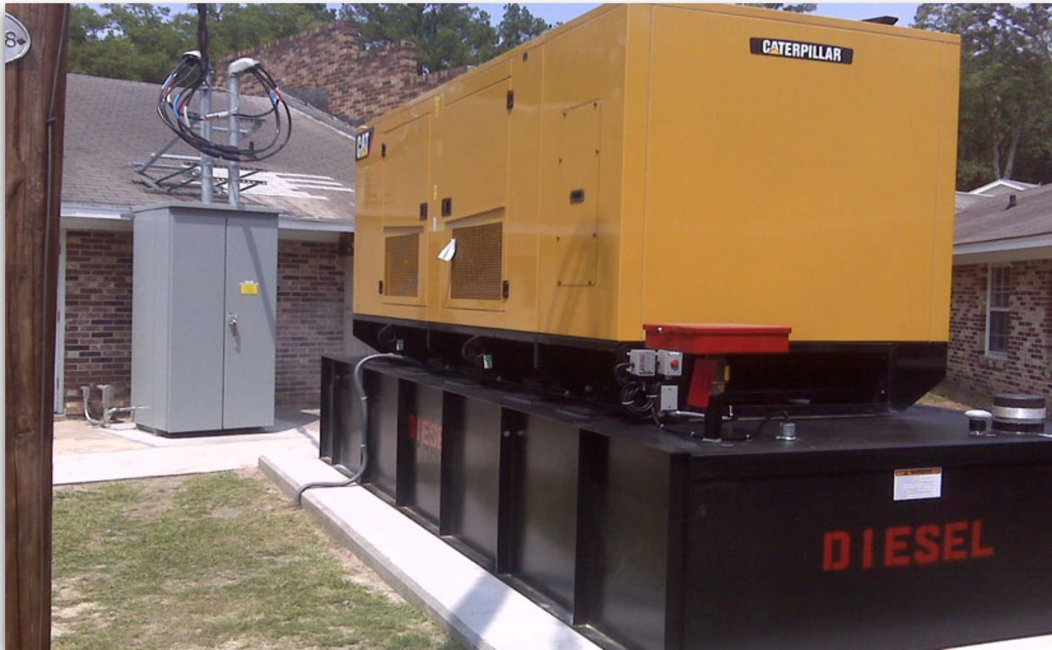
A Caterpillar 20kW packaged diesel generator and automatic transfer switch protecting a small hospital building in the Florida Keys. This is a standby generator, not a UPS.
